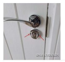
Issue 28 Cloakroom All fixings should be installed to secure the lock
