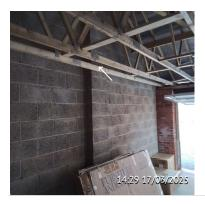
Issue 227 Garage Remove the mortar from the top of the ceiling cord
