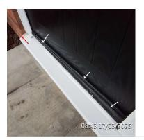
**Issue 7 Front Door** Weatherbar to the front door is scratched and threshold end cap to fully fit
