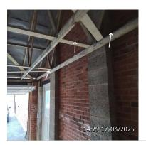
Issue 228 Garage Remove the mortar from the top of the ceiling cord
