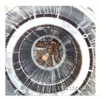
Issue 204 Front Manhole to clean and remove the rubble
