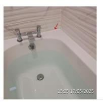
Issue 187 Bathroom Grout to complete to the wall tile
