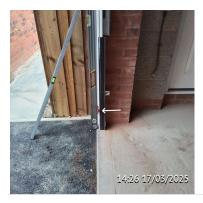
Issue 226 Garage Garage door is out of plumb by 10mm
