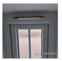
Issue 34 Cloakroom Screws missing from the trickle vent
