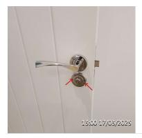
Issue 181 Bathroom All fixings should be installed to secure the lock
