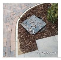
Issue 206 Front Manhole lid to be replaced as damaged
