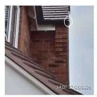
Issue 207 Front Guttering has been finished short to the verge
